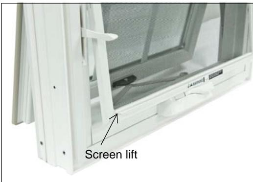
To remove casement/awning screen, grasp screen lift. Lift upward and draw screen towards you, removing screen from channel.
